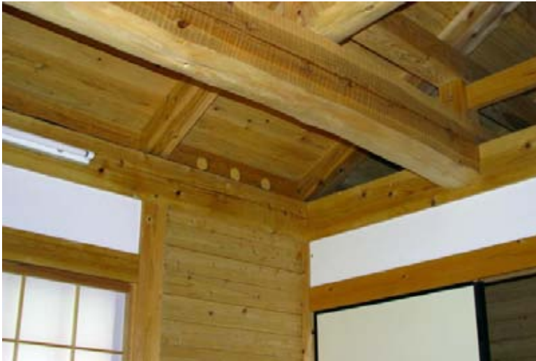
Display house all made from local timber in Miasaki hinterland based on traditional forms combined with energy efficient design. Building design by regional planner and permaculture activist Osamu Matsushita
