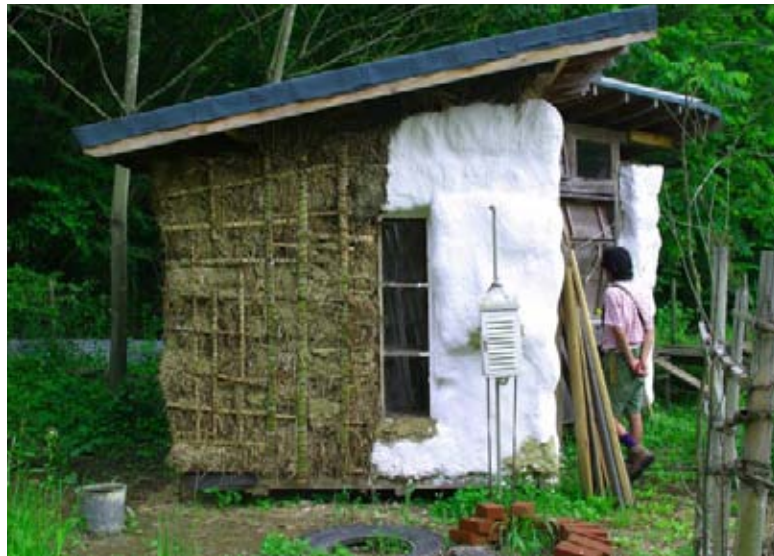
Partly constructed “strawbale” experimental building at Permaculture Centre Japan garden site
