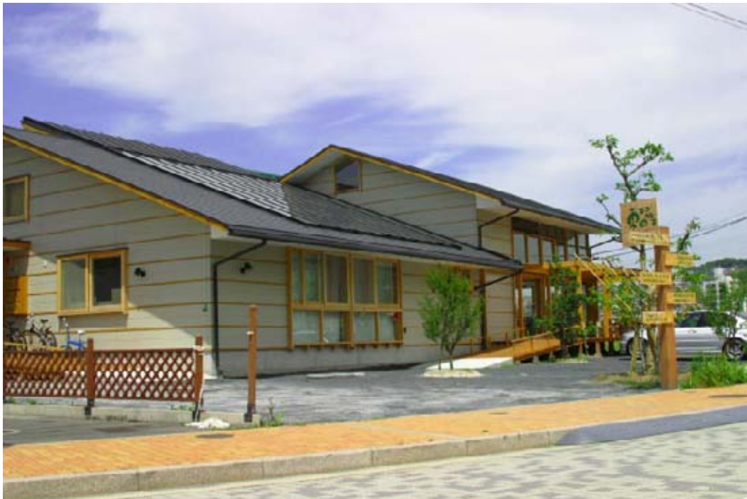
Recently constructed ecological office building Kitikyushu with simplified “OM Solar” roof mounted active air collector supplying thermal mass storage for heating and cooling.
